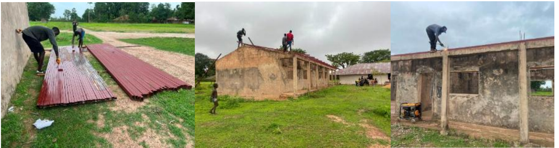
Photos of the renovation of the schools in Patche Ialá and Untché
